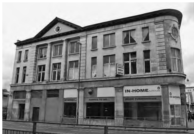
Former Petrol station on Canal Street
